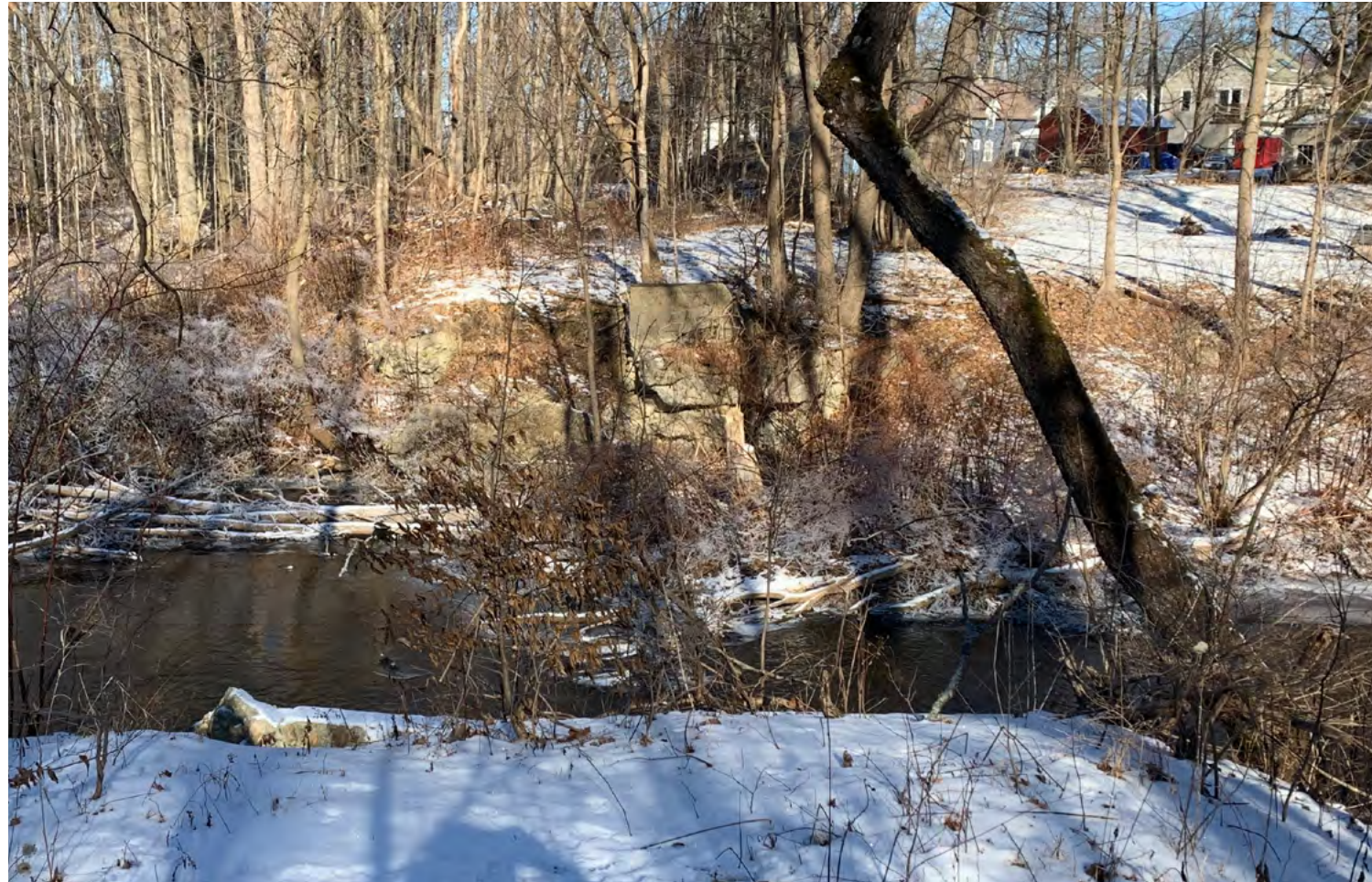
Old trolley bridge abutment in Section 2.
