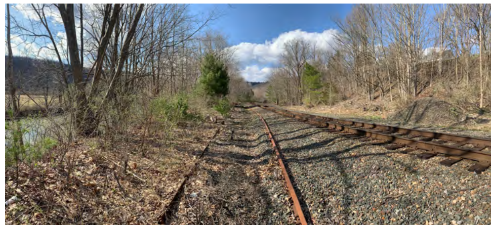
The strip of land between the river and the railroad.
