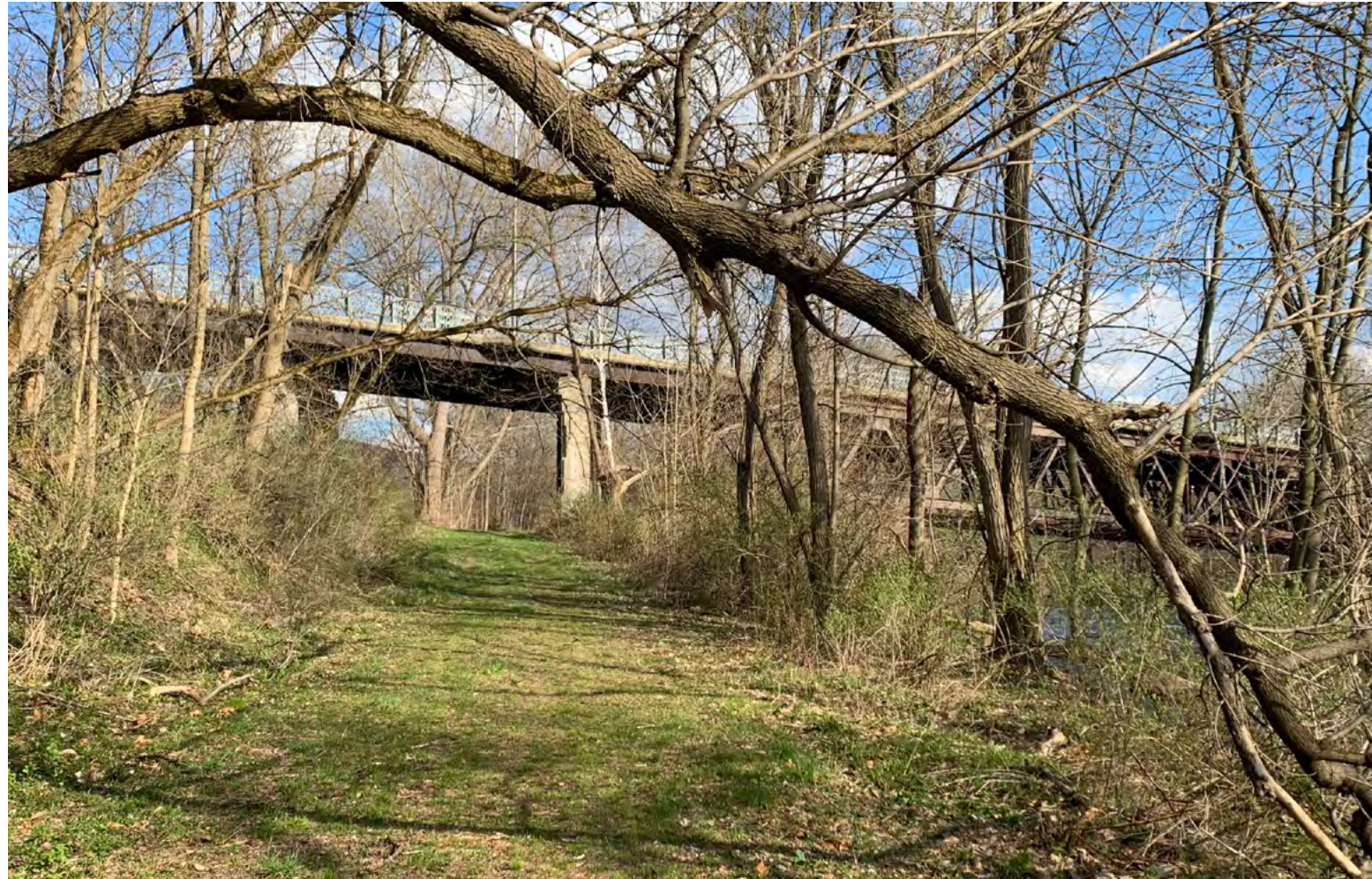
Route 7 Bridge over the Hoosic
