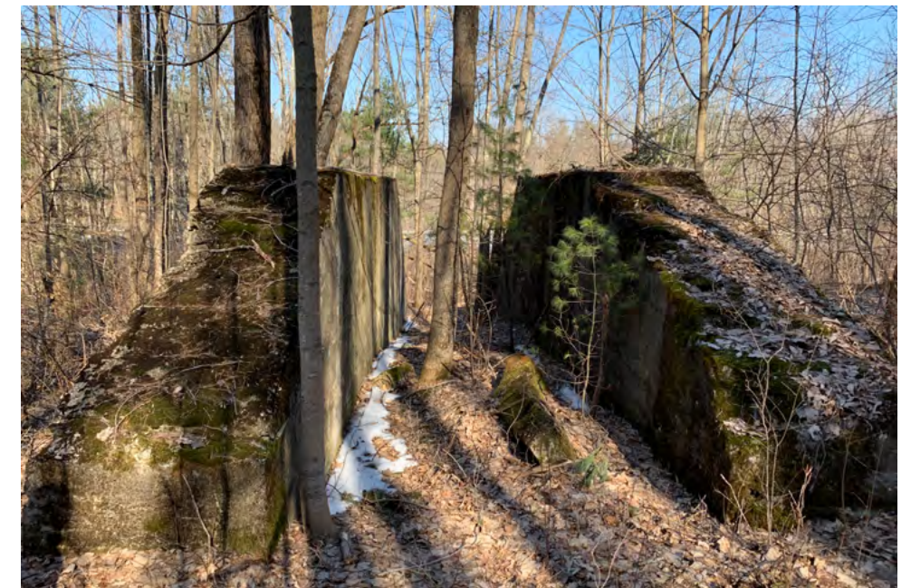
This cattle pass in Pownal allowed livestock to walk under the trolley tracks.
