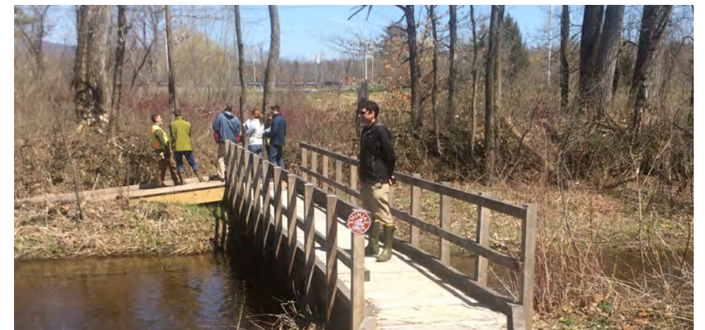
Temporary, low-cost timber bridge constructed by the Town of Bennington for the Ninja Path. It will be replaced with a much larger steel bridge when the federally-funded project is built.
