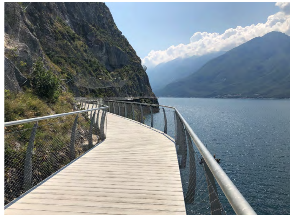
This bicycle path in Italy has made its challenging site a feature.
