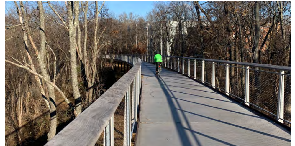
The recently built Neponset River Greenway has elegantly solved site challenges.
