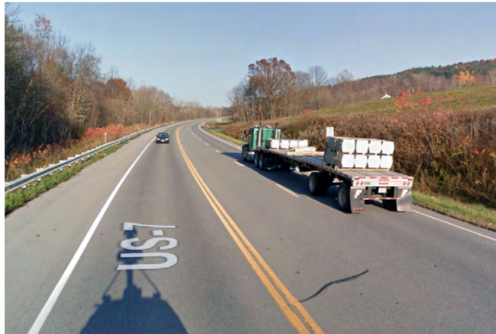
Route 7, between the Massachusetts border and Pownal Center, has some sections with shoulders wide enough for cyclists, but with many large trucks and most vehicles traveling 50-60 mph, it is dangerous and unappealing to bicycle on. Note the narrow shoulder between the truck and the edge of pavement.
