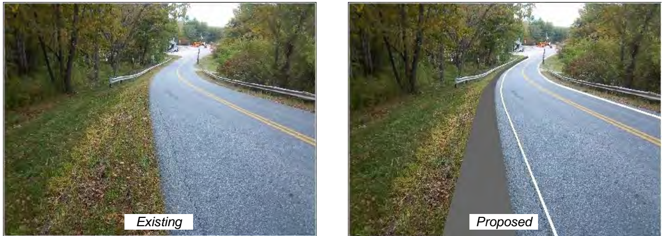
Figure 4-8: Photo Simulation - Paved Shoulder on Sunderland Hill Road (looking north towards Dunham Road)
