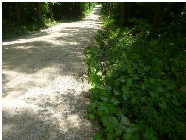
Photo 1: Ditches along Flynn Hollow Road and North Road carry a large volume of sediment.
