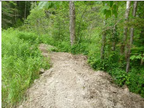
Photo 2: The turnout along the edge of a wetland is buried in sediment.
