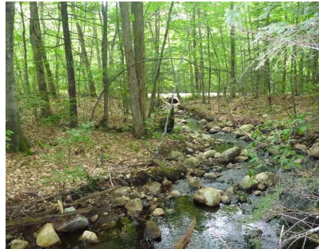
Figure 2: Incised channel upstream of the North Road culvert.
