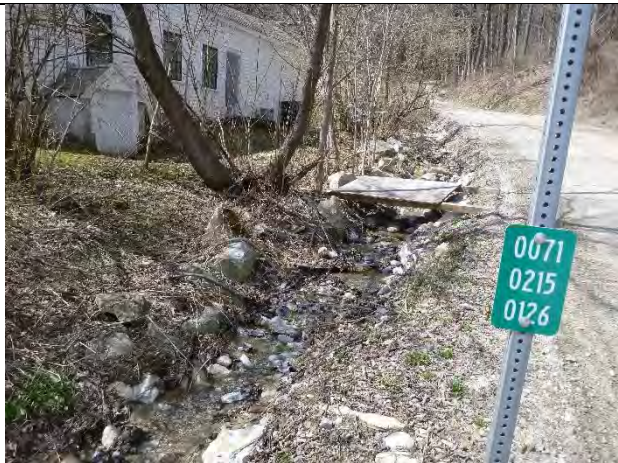
Photo 1: Steep channel approaching the culvert.
