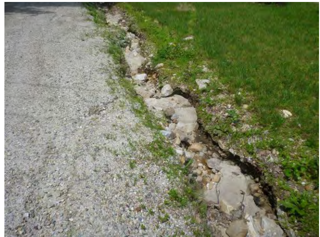
Figure 4: The AOP barrier created by a perched 48" culvert along South Road (left) was the lowest scoring projects (SC-2). The extreme erosion along the edges of Barney Orchard Road (right) was the highest scoring project (RD-8).
