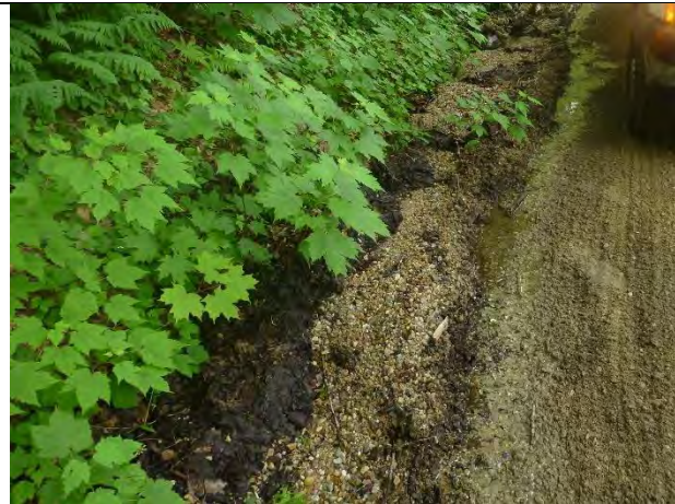
Photo 2: Ditches are filled in along a section of Kelley Stand Road.
