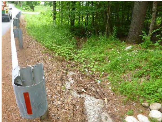
Photo 2: There is space for a BMP between the guardrail and floodplain to treat ditch runoff.
