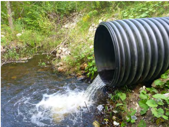
Figure 4: The AOP barrier created by a perched 48" culvert along South Road (left) was the lowest scoring projects (SC-2). The extreme erosion along the edges of Barney Orchard Road (right) was the highest scoring project (RD-8).
