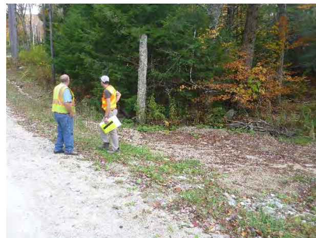
Photo 2: Large turnout to floodplain is filled with road sediment.
