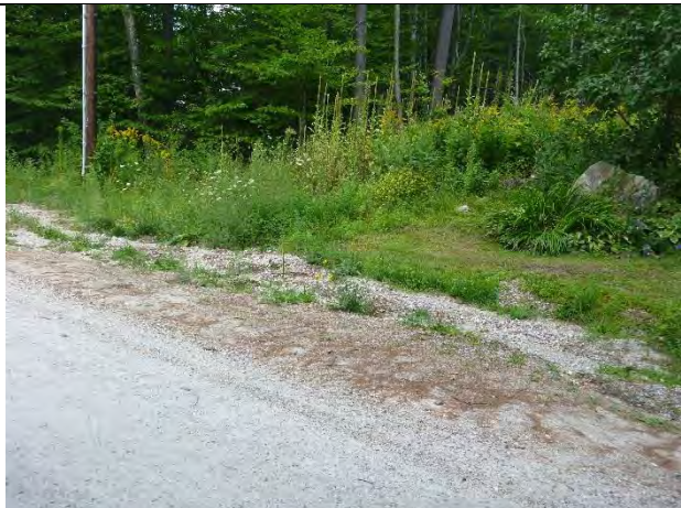
Photo 1: A section of Shady Pines Road has no ditch.
