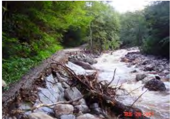
Figure 2: Washout along Kelley Stand Road after Tropical Storm Irene. Photo courtesy of BCRC.
