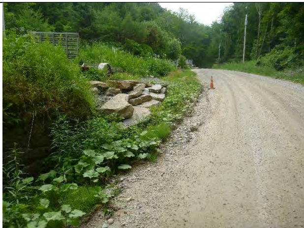
Photo 1: A recently installed driveway culvert along Kelley Stand Road.
