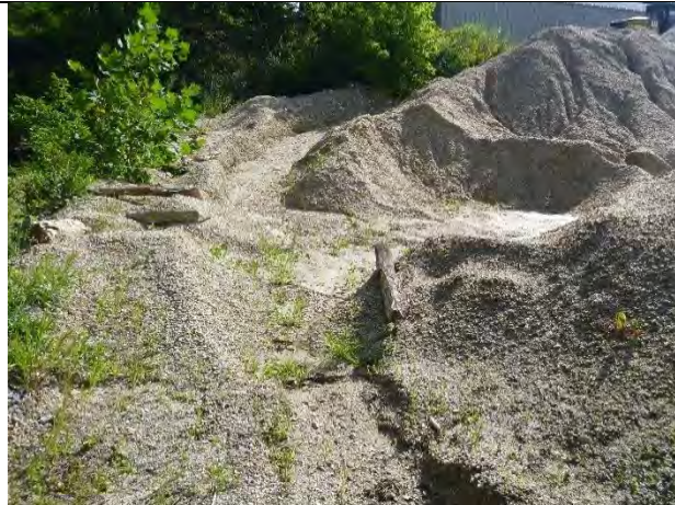
Photo 2: Erosion is overloading the sediment trap.
