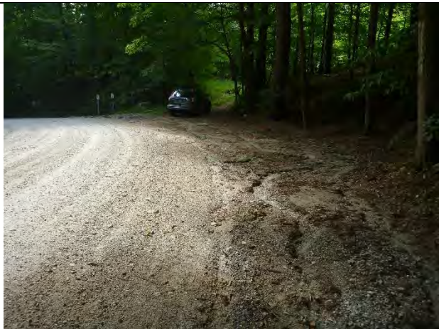
Photo 1: Erosion along Bentley Hill Road.
