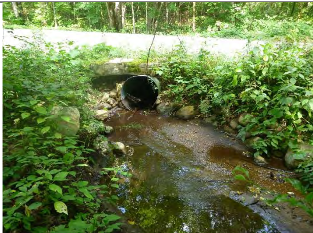
Photo 1: A 36" CMP conveys a small stream under Dunham Road.
