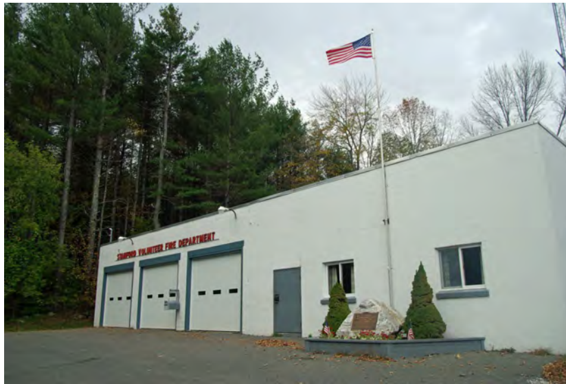
The Stamford Volunteer Fire Department provides a full range of emergency fire, medical, and natural disaster services to the community, operating out of this centrally located facility on Mountain View Lane.
