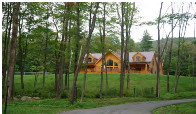
Single family homes on relatively large lots are common throughout much of the Residential District.
