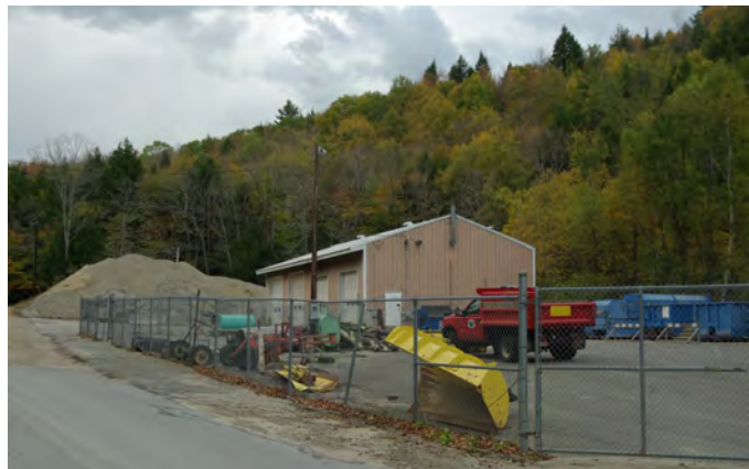
The highway garage also is the site of the Town's transfer station.
