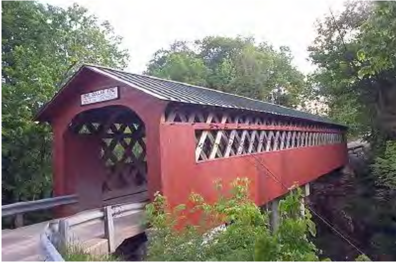
Chisville Bridge, Sunderland
