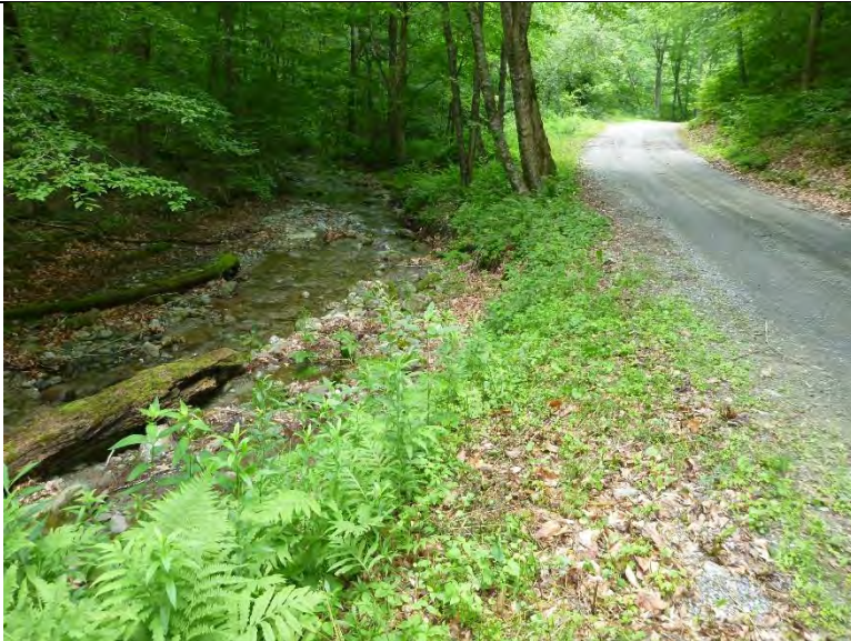
Photo 1: Erosion where Chunks Brook flows alongside the Tate Hill Road embankment.
