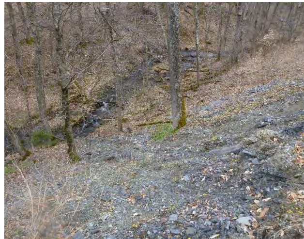
Figure 3: Gully erosion along the steep Rupert Road embankment.
