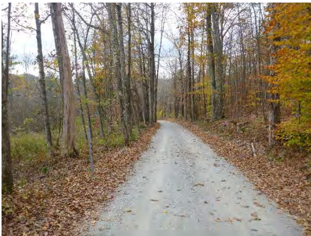
Photo 1: The road has a near continuous tall grader berm (with large trees) along the east side and an undersized and shallow ditch along the west side.
