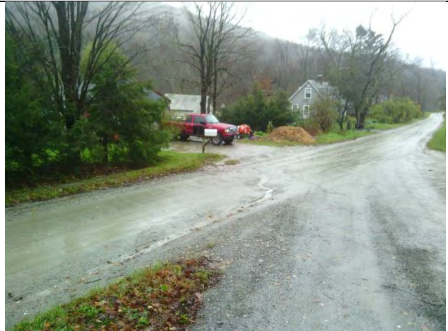
Photo 2: Runoff from Wuerslin Road causing significant erosion as it crosses Sandgate Road.
