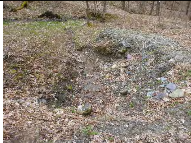
Photo 2: Cross-culvert outlet with gravel dumped alongside channel flowing toward Sandgate Brook.
