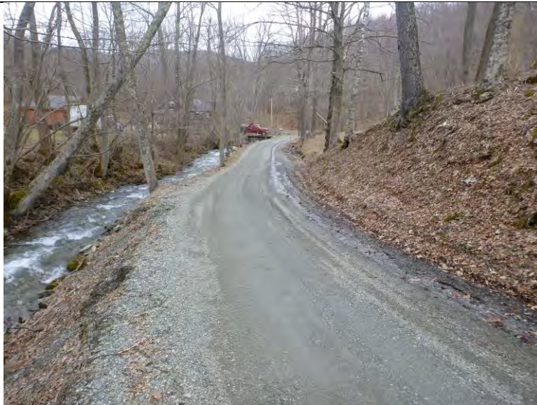
Photo 1: Narrow road with Hopper Brook on left and limited space for a ditch on the east side of road.
