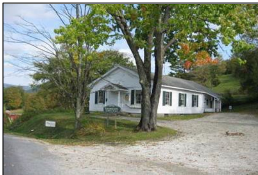
Figure 19: Sandgate Town Office
