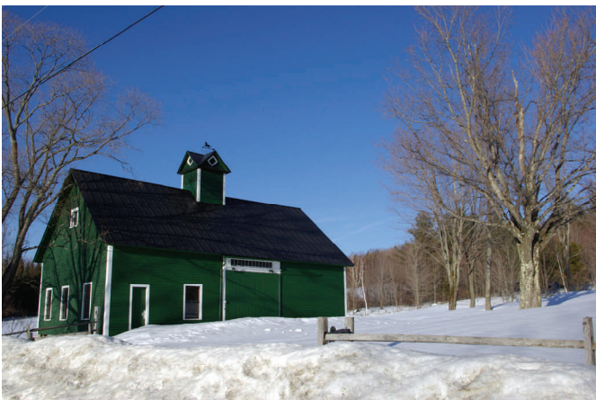
The sharp well-defined edges of buildings and distinctive paint colors can create strong contrast in rural landscapes.
