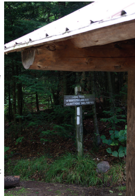
The Peru Peak shelter is located on the AT/LT near Griffith Lake.
