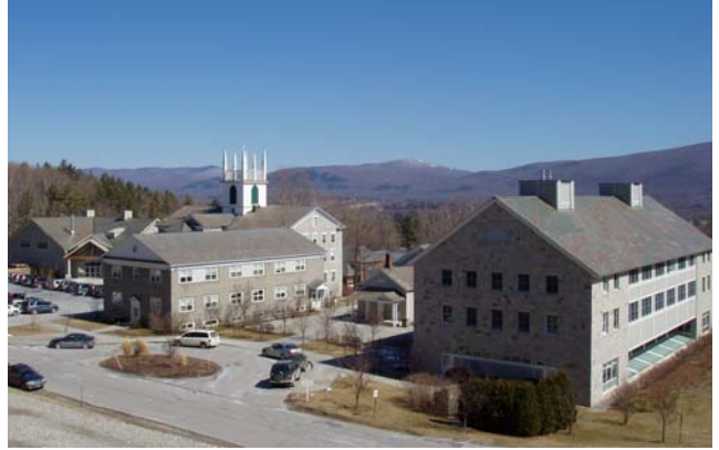
The Burr and Burton Academy campus includes a complex of significant historic and contemporary educational buildings.
