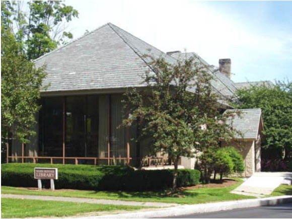
The Mark Skinner Library is an important historic structure that occupies an extremely prominent location in the center of the Village.
