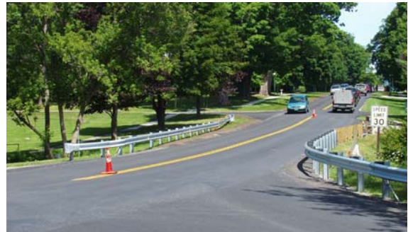
Roadway projects should be sensitive to the scenic character of surrounding landscape. In this case, roadway width has been maintained, but the design and expanse of the guardrails at important entry to the Village could have been improved.
