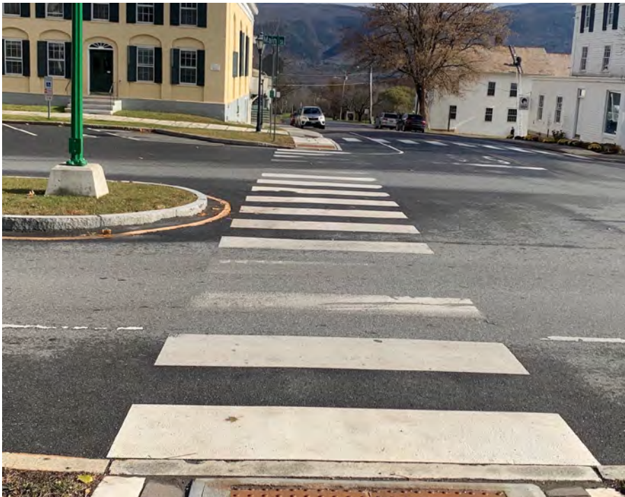
Existing condition: pedestrians crossing Route 7A in front of the Equinox are exposed to traffic for a long distance.
