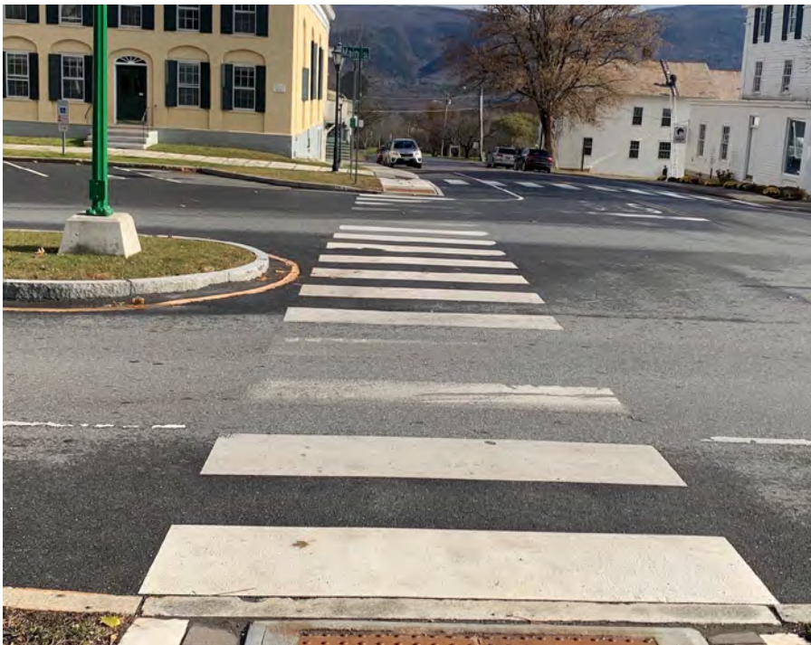
Existing condition: pedestrians crossing Route 7A in front of the Equinox are exposed to traffic for a long distance.
