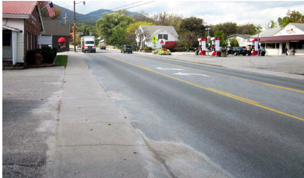
Depot Street has wide expanses of pavement and lacks street trees.
