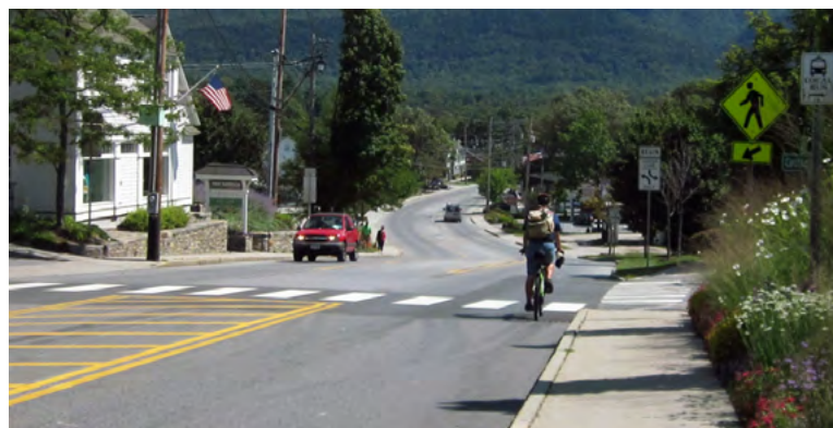
Hill on Depot Street. Cyclists travel closer to the speed of traffic going downhill. Shared lanes are safer than bike lanes on downhill grades.
