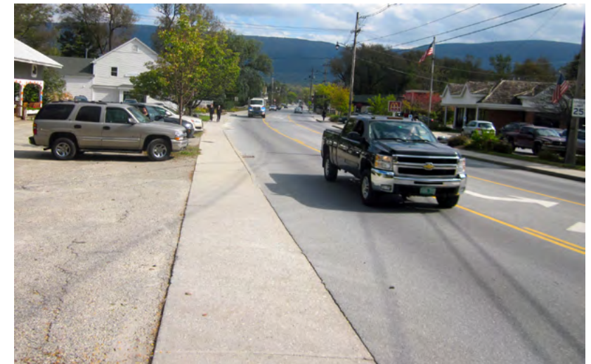
Wide driveway access near Manchester Woodcraft
