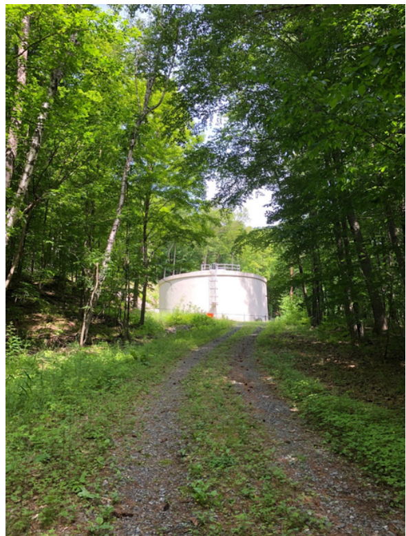
Water tower view from Ursa Way
