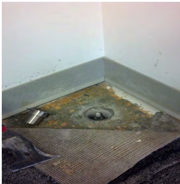
Figure 2: Final sub-slab installation appearance of the Vapor Pin®
