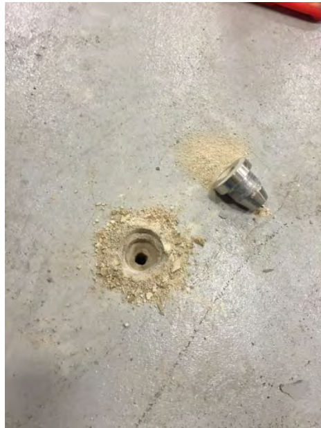
Figure 1: Two-staged sub-slab drilling for the installation of the Vapor Pin®
