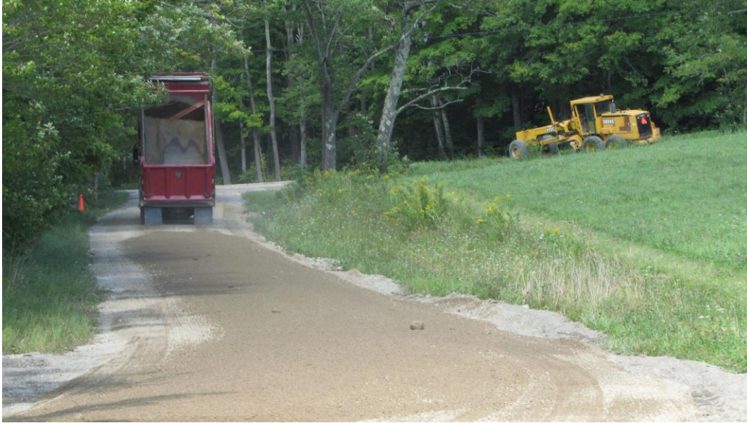
Road Work on Upper Hollow Rd
