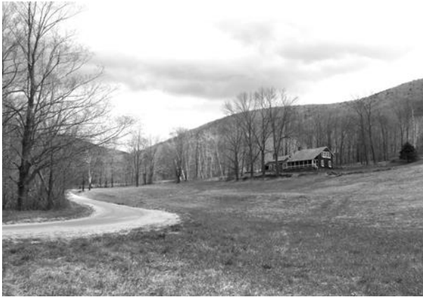
3A. The access to this house follows the treeline and then rises following the natural contours of the land, preserving the visual appeal of the open field in the foreground.
