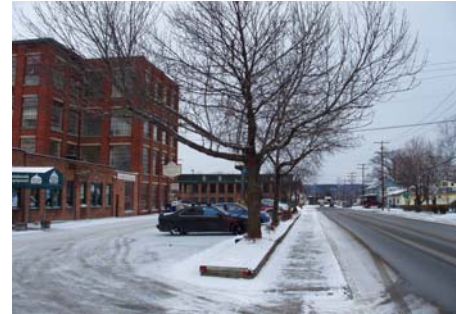
Reuse of historic buildings is a central objective of the UMU District.
