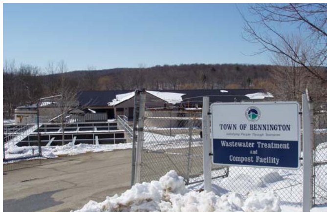
The municipal wastewater treatment plant includes an innovative sludge composting facility.
