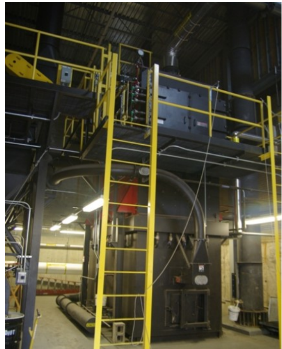
Forests cover most of Bennington County; the wood available from Bennington County and surrounding areas can provide energy for facilities such as this 400 horsepower wood boiler system at Bennington College, which has reduced oil consumption on the campus by more than 300,000 gallons per year.
