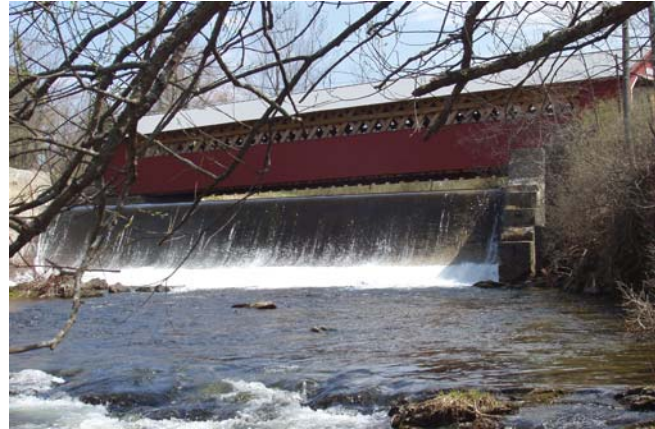
Many of Bennington’s historic structures are located along its waterways, such as the three covered bridges over the Walloomsac River.
