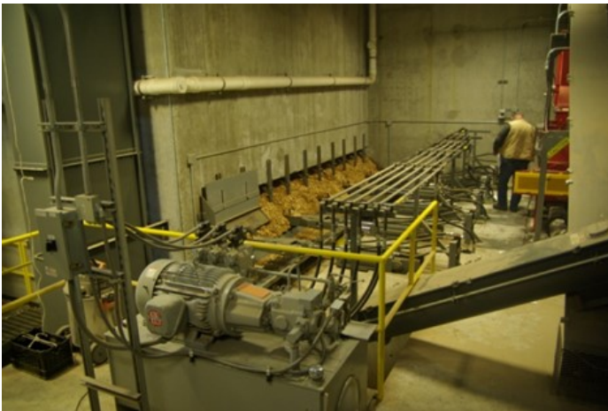
Forests cover most of Bennington County; the wood available from Bennington County and surrounding areas can provide energy for facilities such as this 400 horsepower wood boiler system at Bennington College, which has reduced oil consumption on the campus by more than 300,000 gallons per year.
