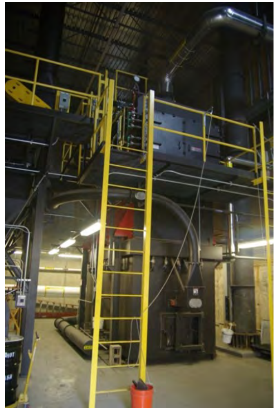
Forests cover most of Bennington County; the wood available from Bennington County and surrounding areas can provide energy for facilities such as this 400 horsepower wood boiler system at Bennington College, which has reduced oil consumption on the campus by more than 300,000 gallons per year.
