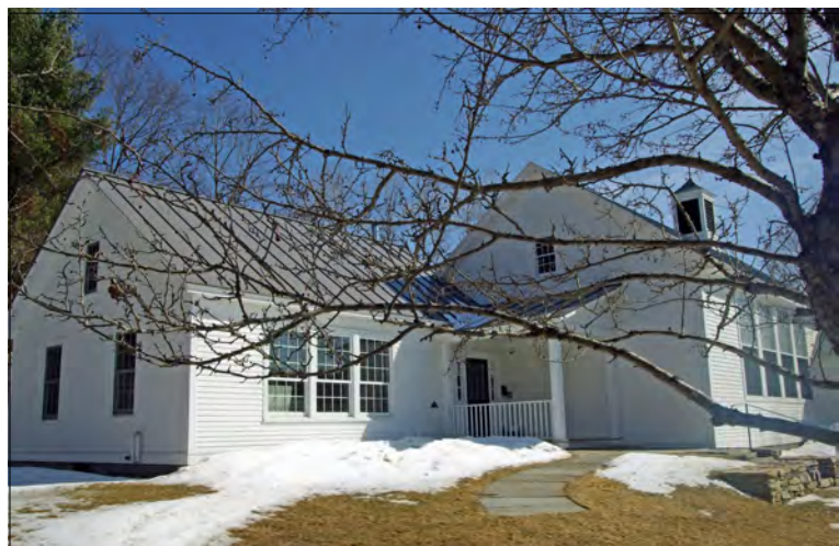
A new addition to the Landgrove Town Hall has made that building more comfortable and efficient.
