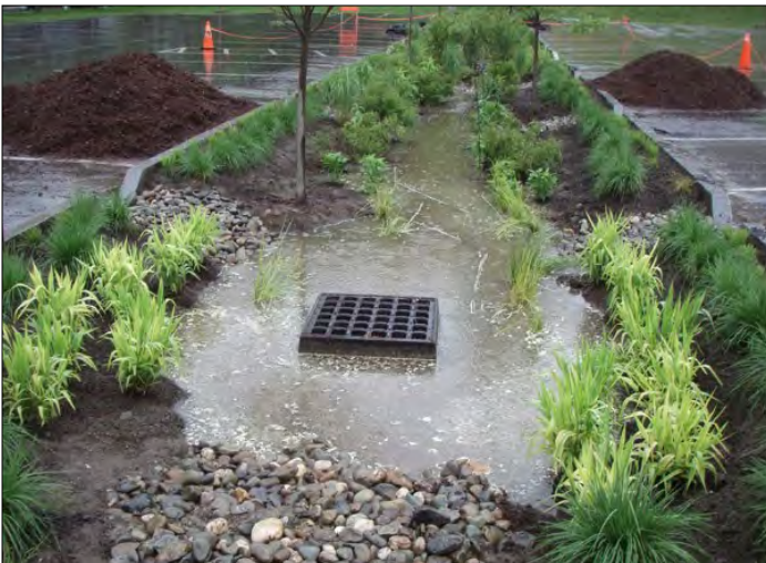
Towns and villages can require rain gardens (shown above) and other stormwater management strategies that capture, slow, infiltrate, and treat runoff from impervious surfaces, including rooftops, streets, parking lots and driveways.
