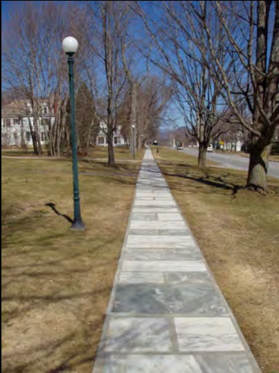
Reconstructed marble sidewalk in Manchester village.
