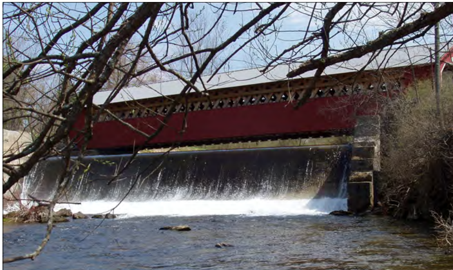
The owner of the “Paper Mill” dam and former mill building on the Walloomsac River in Bennington is re-establishing hydroelectric generation at the site. A similar project is planned for the former tannery dam in Pownal. Other sites having high potential for hydroelectric development in the region include the dam at Lake Paran and the four Paran Creek dams in North Bennington, and the dam on the West Branch of the Batten Kill in Manchester.
