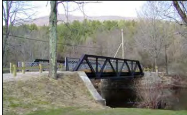
This historic pony truss bridge over the Batten Kill has been preserved and reused at a fishing access site.
