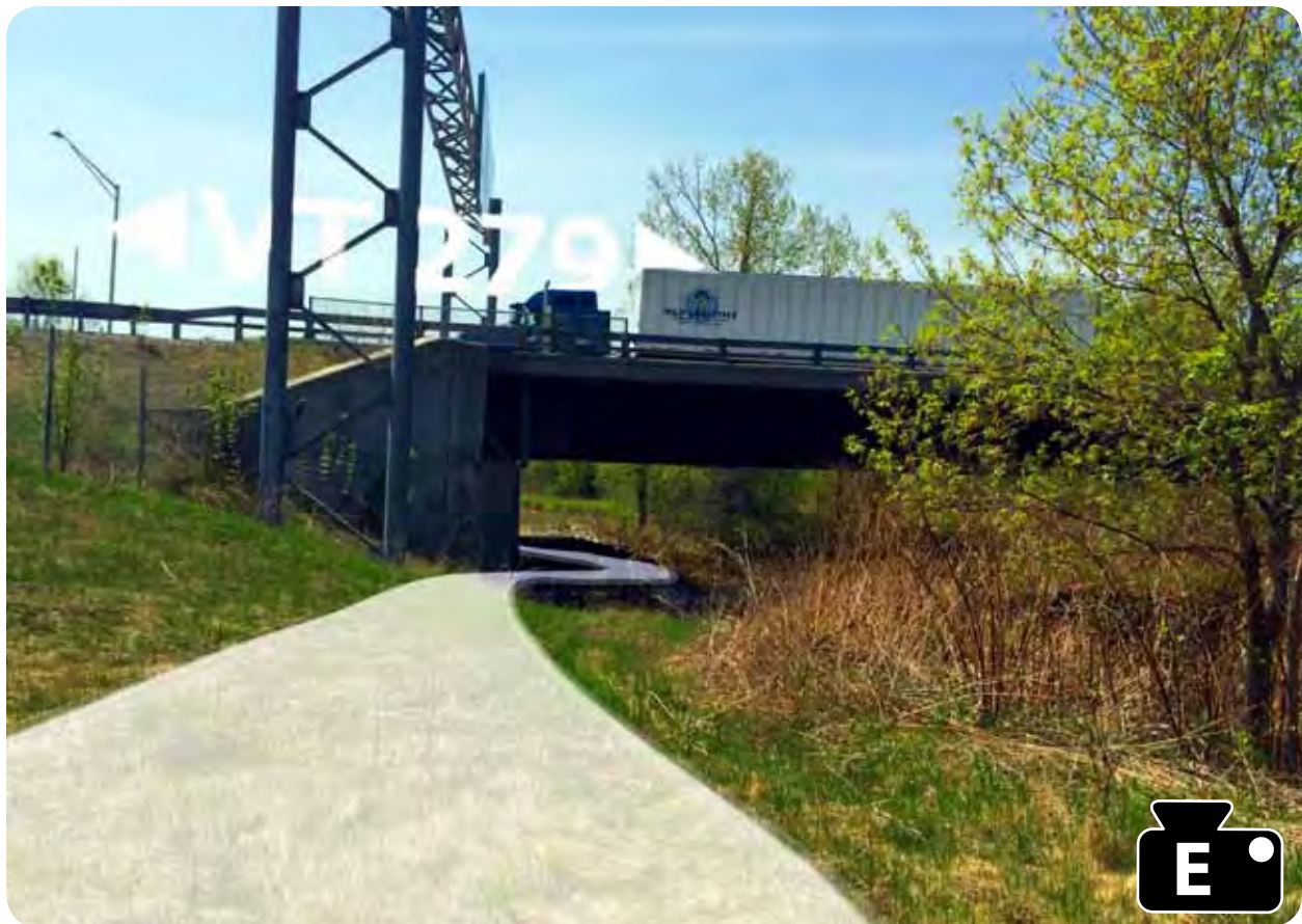
VT Route 279 Crossing: The path will cross under the Route 279 overpass west of the Bennington Visitors' Center and the Route 279/ Route 67A interchange.
