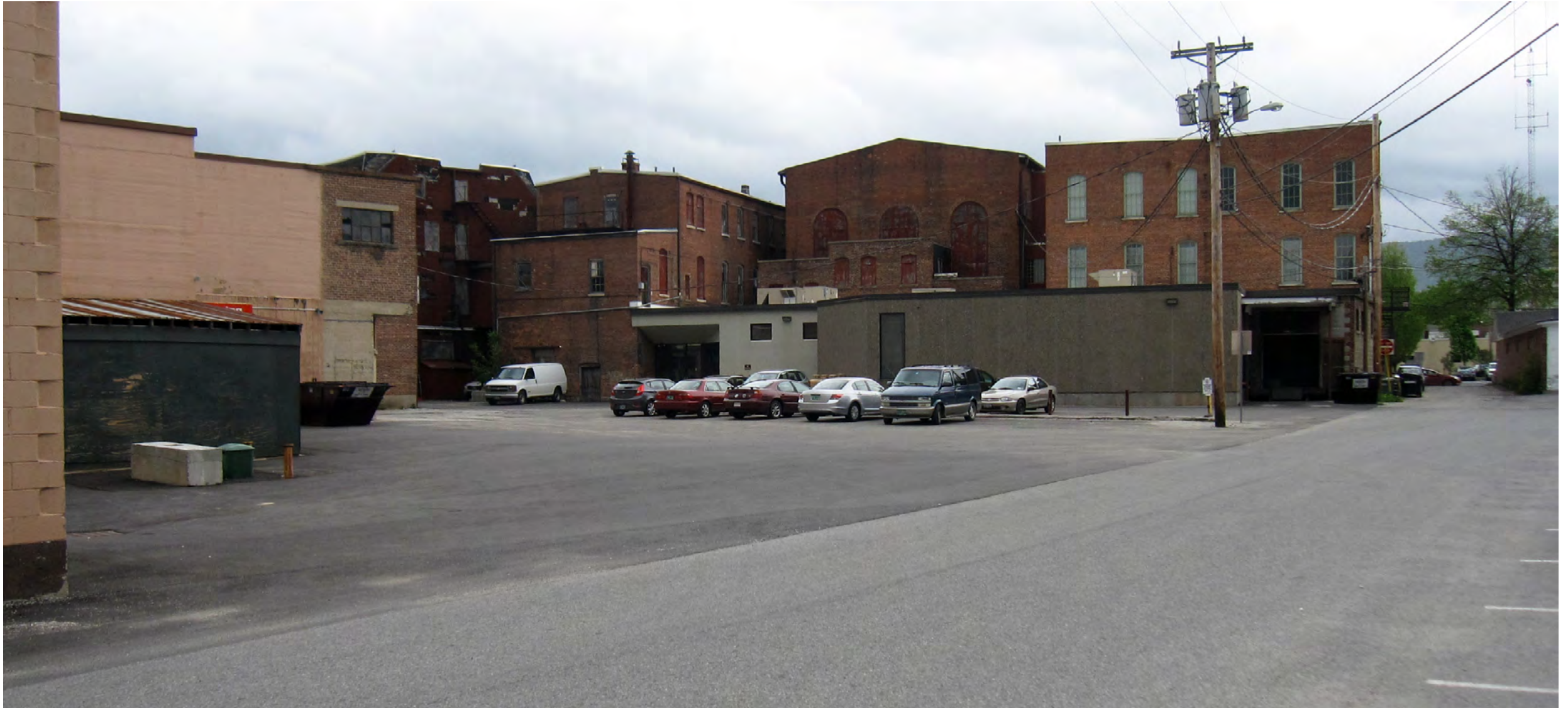
The project area's unbroken expanse of blacktop is visually oppressive. The street lacks definition along its northern edge.
