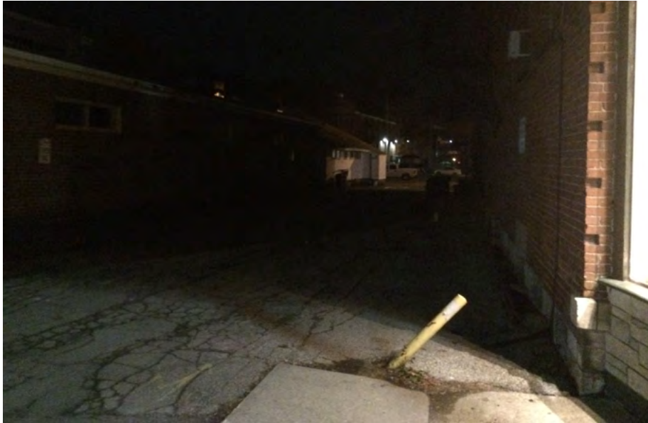
The alley is poorly lit and very dark at night.
