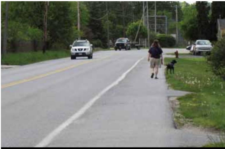
Pavement: There is enough existing pavement to accommodate nearly all of the needed improvements.
