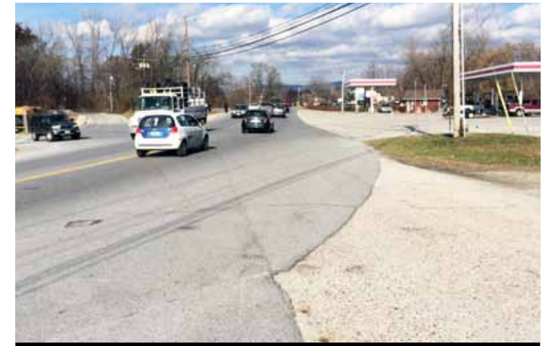
Dangerous Conditions: Sections of Benmont are unsafe for vehicles, pedestrians, and cyclists.
