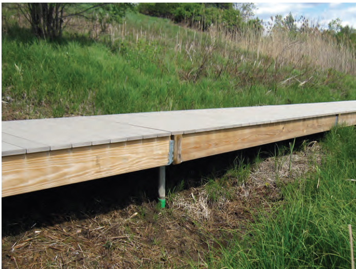
Helical piles support the Paran Pathway in North Bennington.
