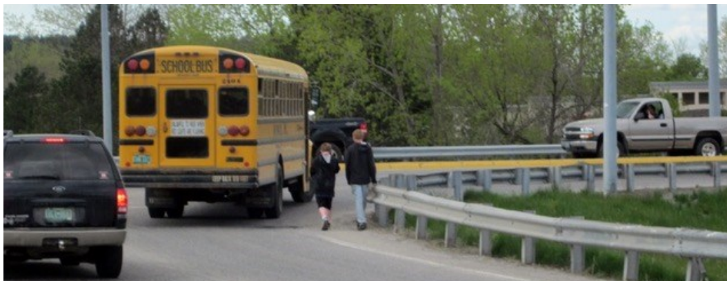
Residents will soon be able to walk and bike safely along the busy Kocher Drive corridor between Benmont Avenue and Park Street, with a safe crossing of US Route 7.
