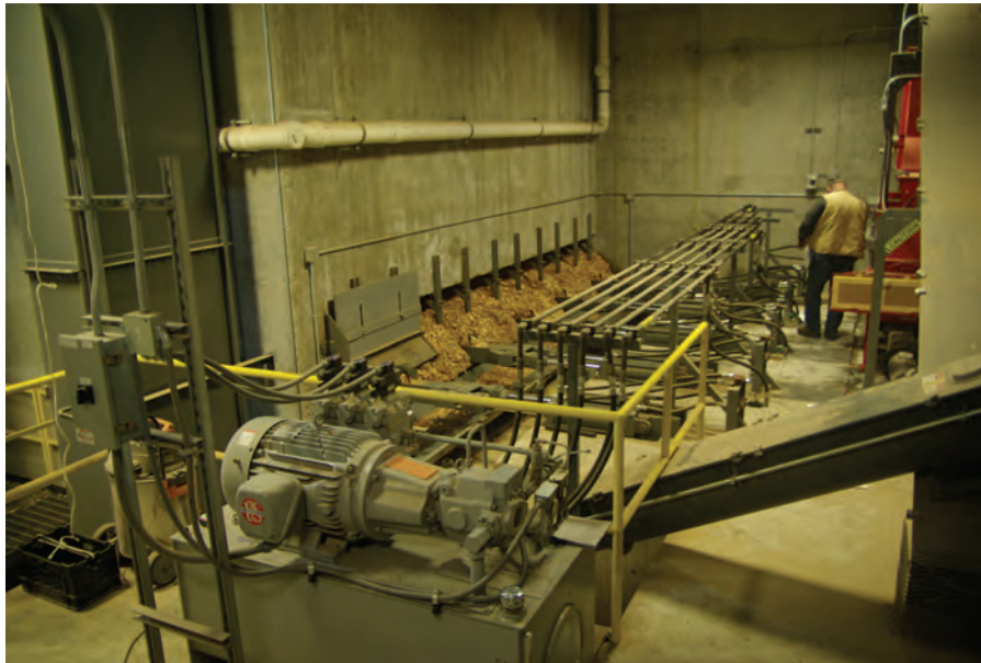
Part of the wood chip based heating system in use at Bennington College.
