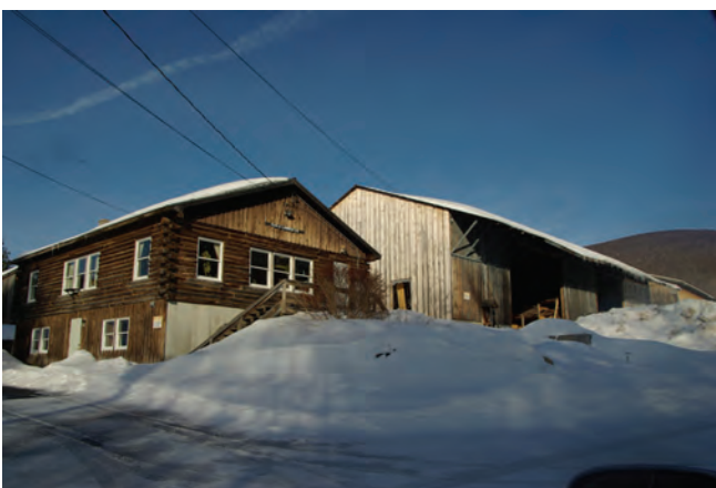
Eagle Lumber in Stamford is one of the few primary industrial users of forest products located in the region.
