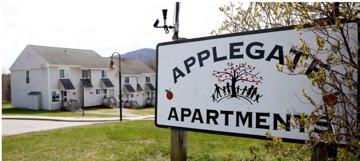
As seen by the examples listed in Table 4.2 , there are a variety of locations in the region that have the potential to save money and energy by converting to biomass district heating systems. Applegate Apartments in Bennington, which is owned by Housing Vermont, plans to link their 104 housing units with a new biomass district heating system. They anticipate saving approximately 50% of current heating costs annually.
