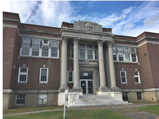
Part of the Benn High building will be redeveloped into housing with CRRP grant funds.
