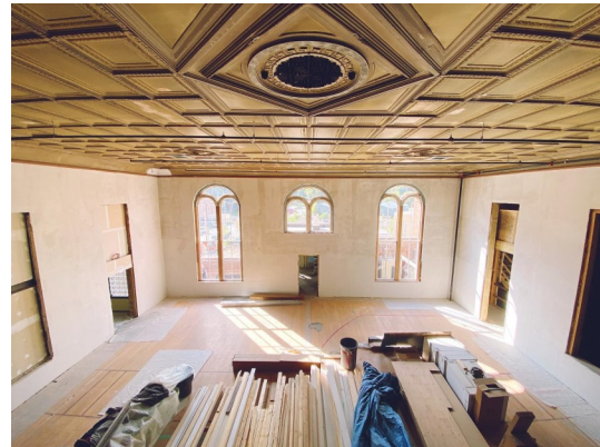
Progress on restoration of interior spaces in the Putnam Block project.
