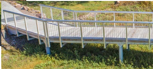
This make-shift path will be replaced with a fully-lit boardwalk and gravel path that will allow children residing at Orchard Village a safe route to walk to the Molly Stark School.
