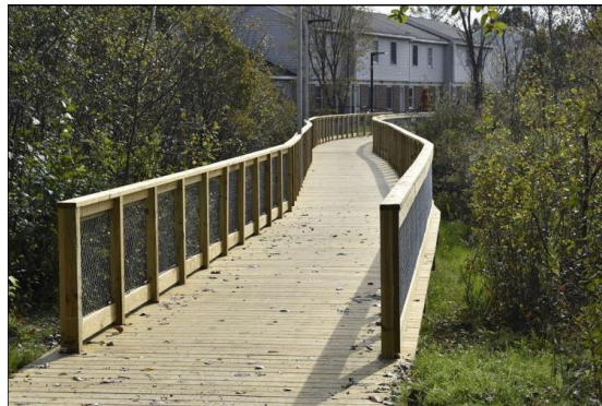
Completed Orchard Village-Willowbrook Path
