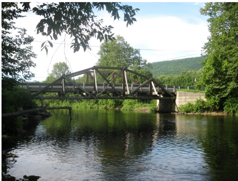
Benedict Hollow Bridge over the Batten Kill in Arlington
