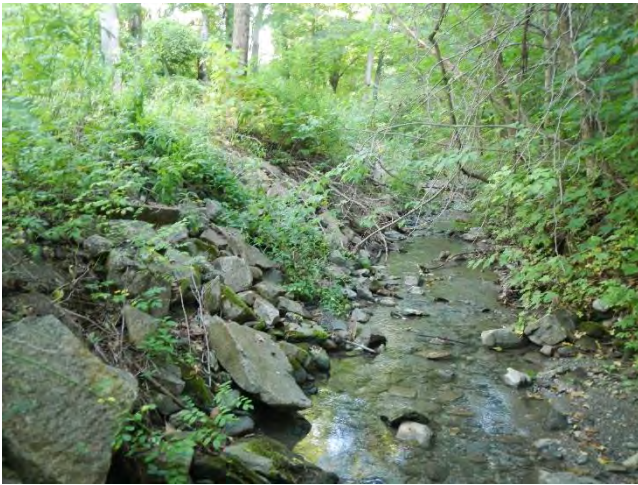
Figure 4.11: Bank armoring pinching channel along Mt. Anthony Road on segment M01T1.04C.
