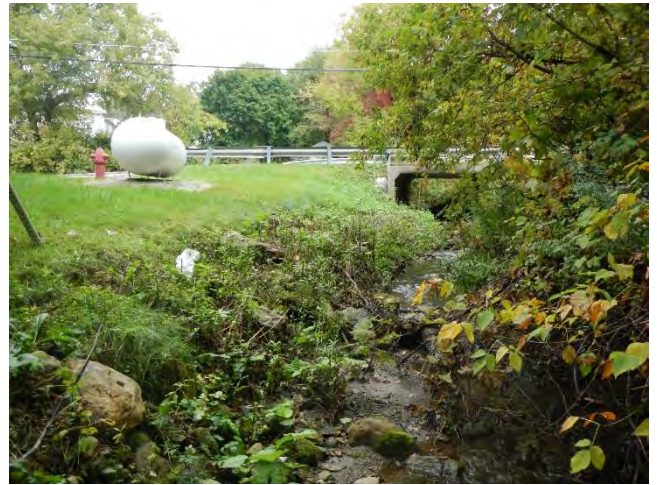
Figure 4.12: Church Street bank armoring in reach M05S1.01.
