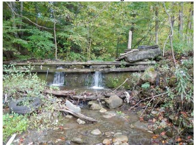
Figure 4.10: Small concrete dam in reach M05S1.02.
