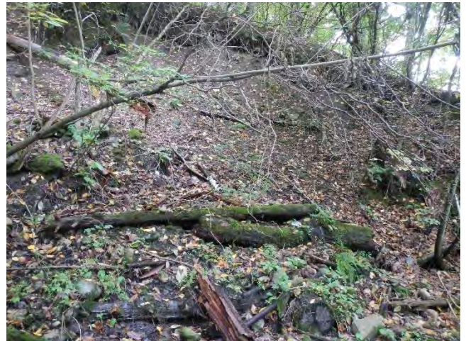
Figure 4.16: Mass failure on reach M05S1.02.
