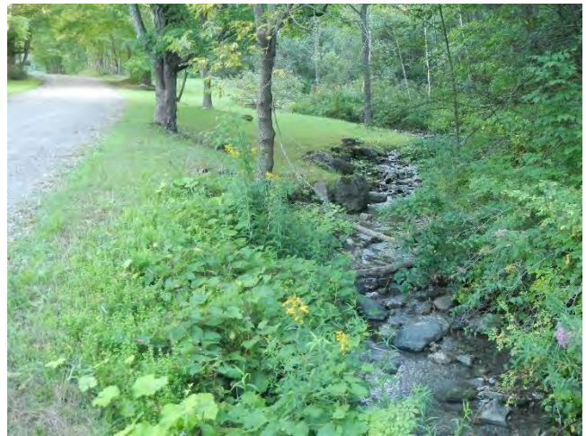
Figure 4.22: High encroachment along Mt. Anthony Road on reach M01T1.04C.
