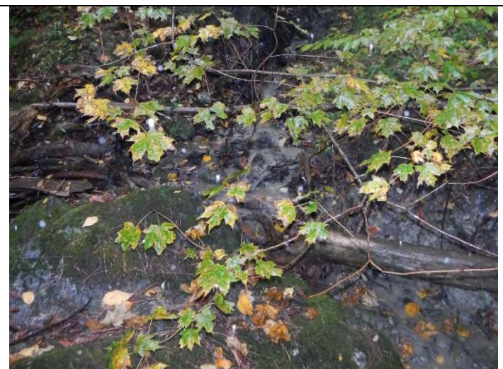
Stormwater runoff from Hemlock Hill Road
