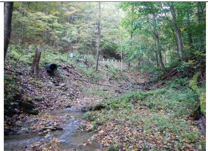
Stormwater outlet and steep embankment along Ladd Rd
