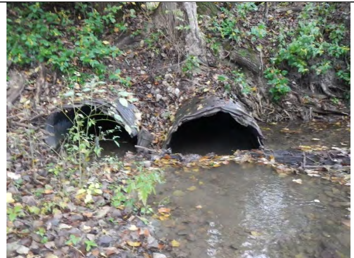
Constrictions affecting channel drainage
