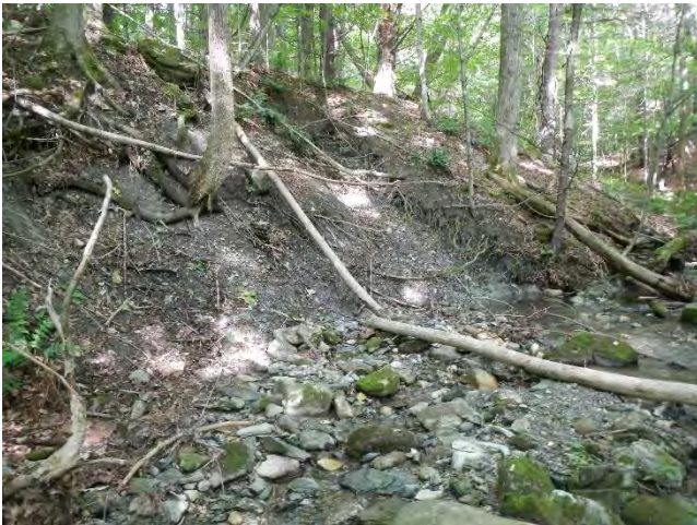
Figure 4.15: Mass failure on reach M01T1.04C.
