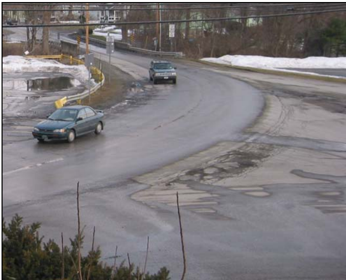
Figure 1: VT 67A-River Road-Hillside Street Intersection
