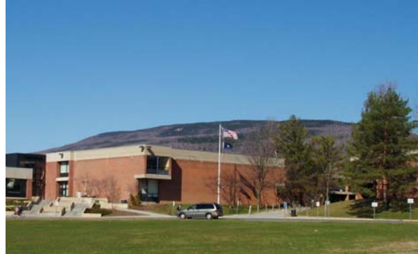
The Green Mountains add visual interest to important public buildings such as Mount Anthony Union High School.
